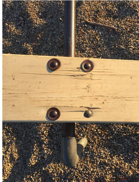
*Figure 30: Deteriorating Playground Equipment*
