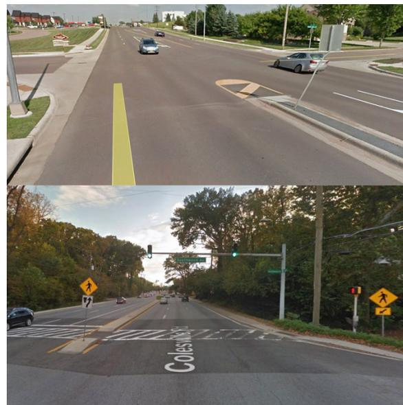
*Figure 25: Current W 69th St. Intersection (top) and example of recommended crosswalk implementation (bottom).*
