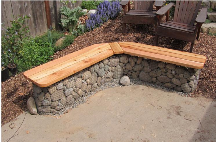
*Figure 26: Gabion bench as a low-cost seating solution*
