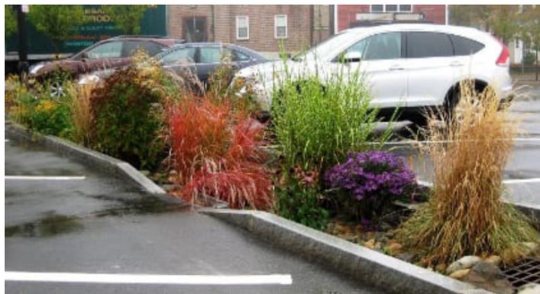
Figure 6: A bioswale acting as a parking lot buffer
